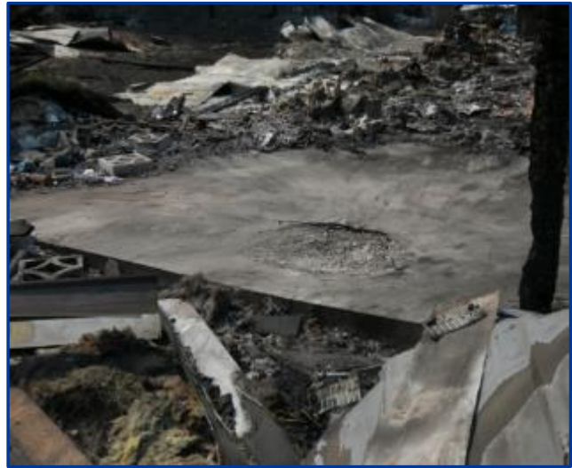
The crater in the concrete pad that resulted from the shed explosion.
