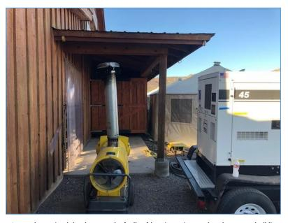
It was determined that because the (yellow) heating unit was placed next to a building with an overhanging roof, the unit's exhaust was trapped and cycled back into the unit's air intake, which was then pumped into the Medical Unit yurt with warm air. The yurt is seen on right in the distance; the generator is on right in foreground.
