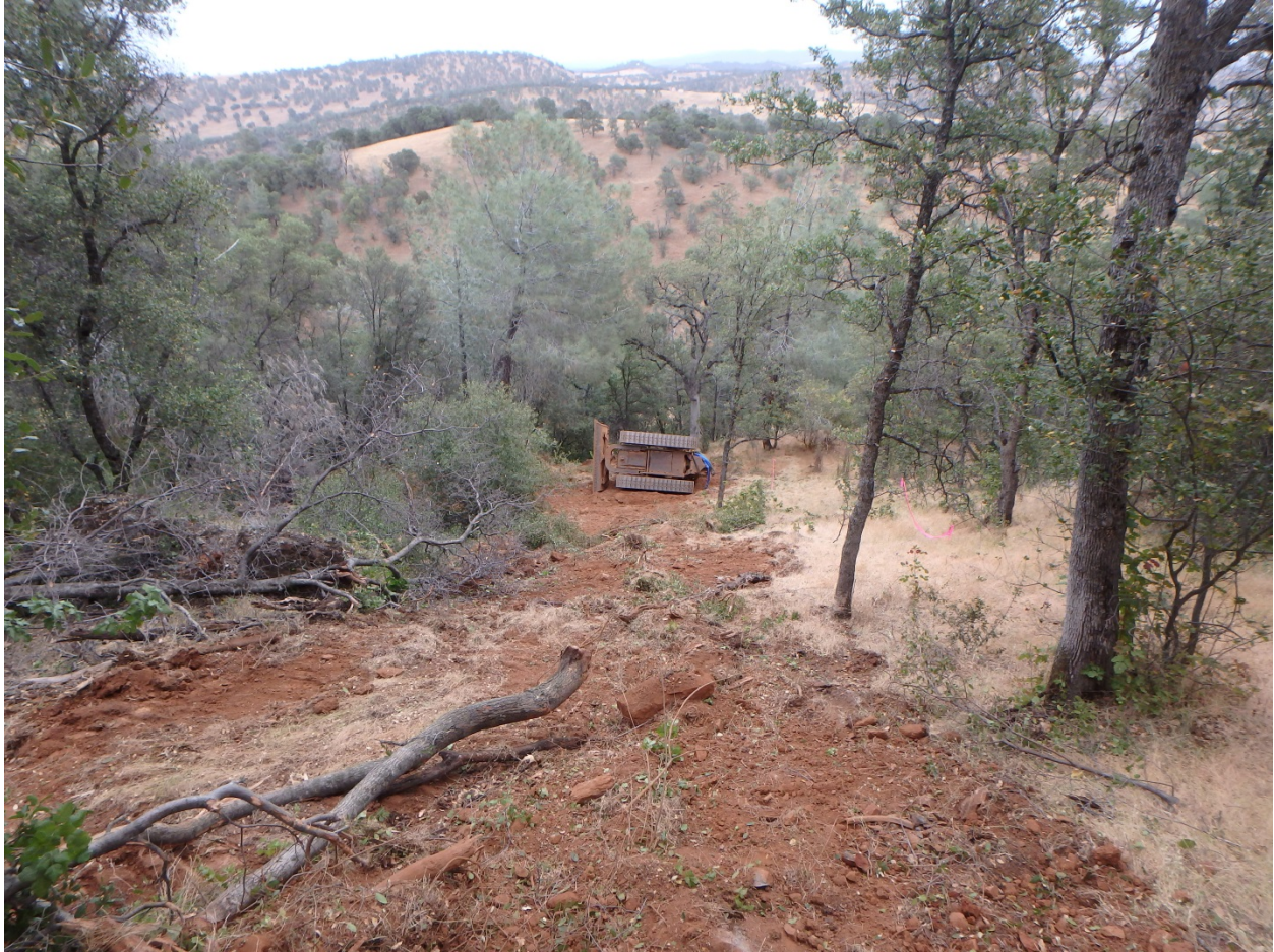
View of D3140 looking downslope on the partially constructed dozer line. Prevailing slopes in this location measured by clinometer at 40%.
