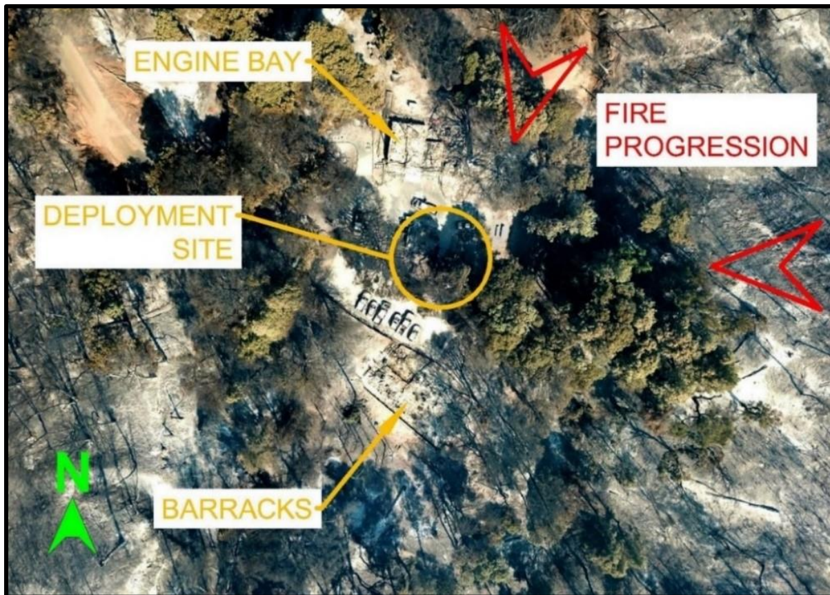
Figure 4. Post-fire overhead view of the Nacimiento compound.
