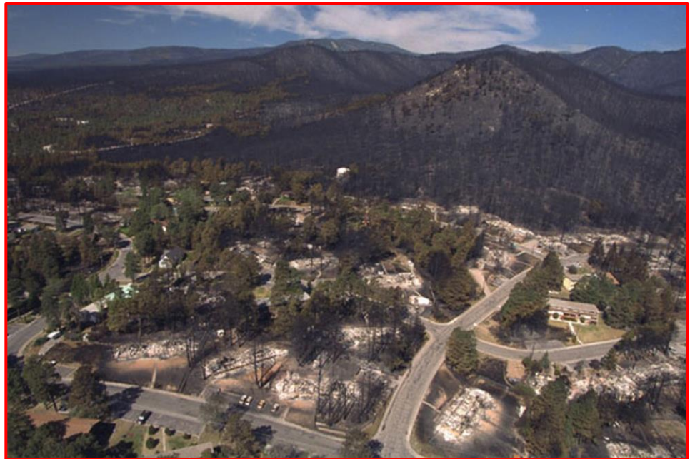
This photo shows some of the more than 230 homes that were destroyed by the Cerro Grande Fire.
